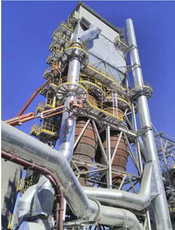
Four-storey coal mill structure.
